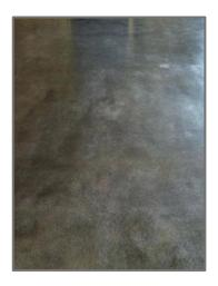
We recommend that the slab is **MACHINE TROWELLED SMOOTH** and even, right to the edges - any 'swirling' or colour variations from the trowelling will remain. This process requires the services of **high quality concretors**. We require a much more dense and consolidated surface for this finish.
